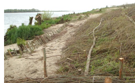
Figure 2 Application of willows for shoreline protection (Image Markus-Michalczyk)
